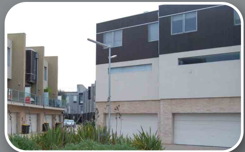
Strata & Public Area Lighting
