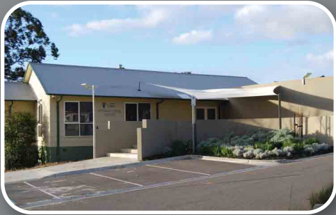
Security and Entrance Lighting
